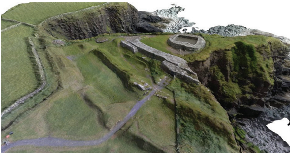
Caer Dunbeg mewn 3D. Roedd y safle eisoes wedi'i ddifrodi gan erydiad arfordirol gan i ran ohono gwmpo i'r môr ar ddechrau 2014. Caiff ei fonitro'n rheolaidd bellach fel rhan o prosiect CHERISH. / Dunbeg Fort in 3D. The site had already been damaged by coastal erosion, with a section of it collapsing into the sea in early 2014, and will now be subject to regular monitoring as part of CHERISH.
