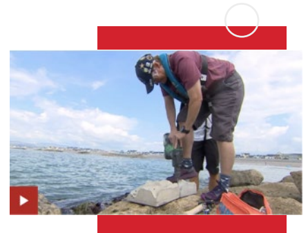
Dr. Pippa Moore attaching an Ecostructure tile to a breakwater in Wales, filmed by BBC News.
